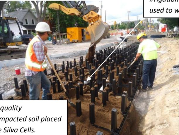
*High quality uncompacted soil placed in the Silva Cells.*
