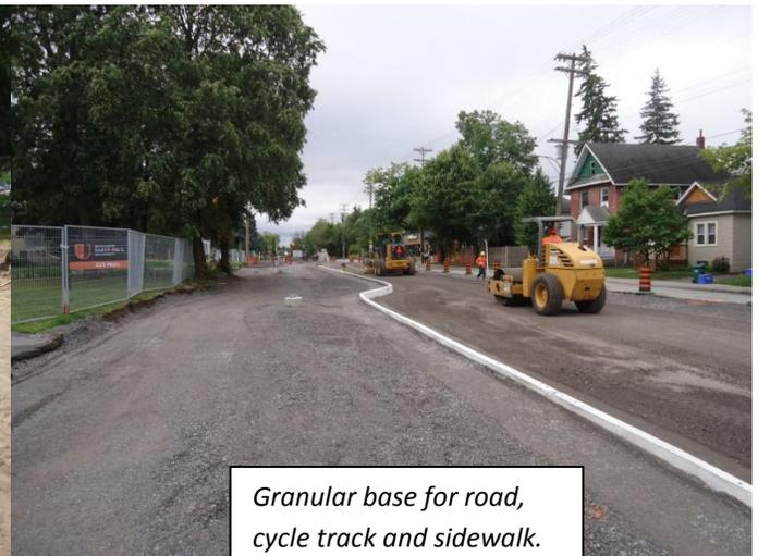
*Granular base for road, cycle track and sidewalk.*
