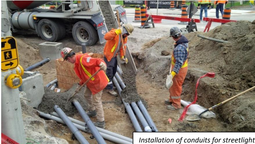
*Installation of conduits for streetlighting and for traffic signals.*
